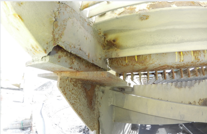
Broken welding on the catwalk of a mill
